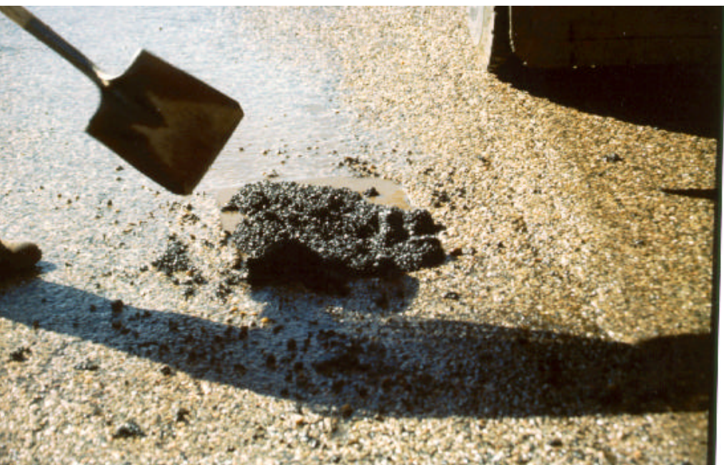
Figure 1. Throw-and-roll procedure—material placement.
