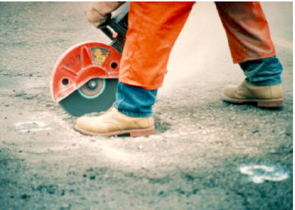
Figure 3. Semi-permanent procedure—straightening edges using hand-held pavement saw.
