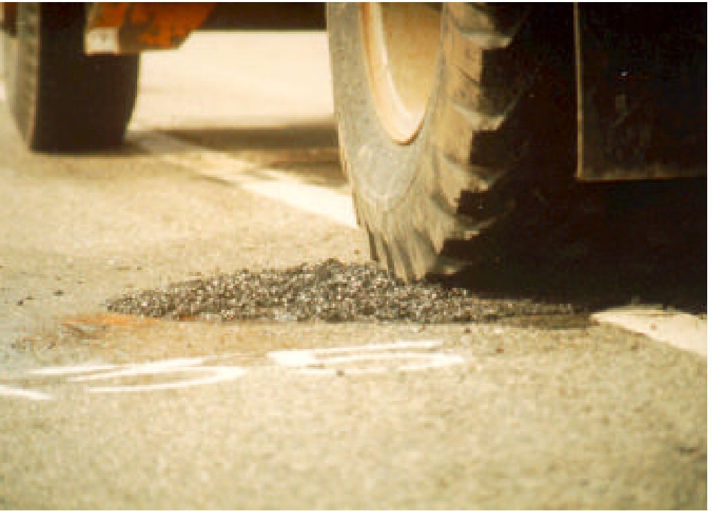
Figure 2. Throw-and-roll procedure—compaction of patch.
