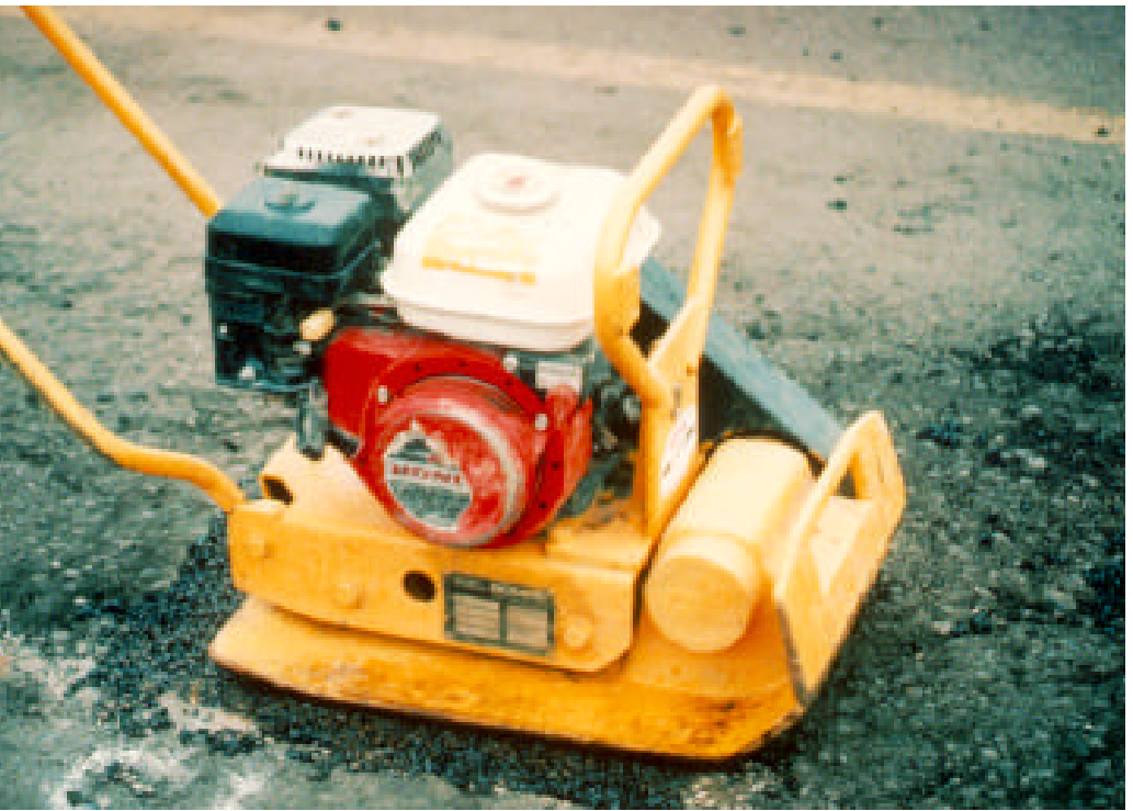
Figure 5. Semi-permanent procedure—compaction using vibratory-plate compactor.
