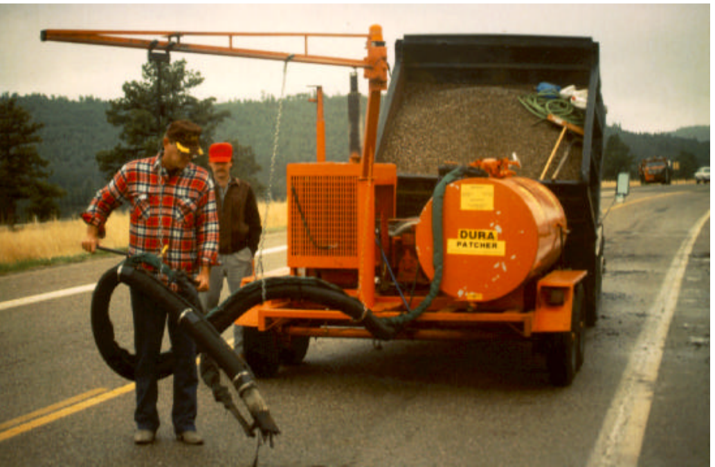
Figure 7. Spray-injection device—truck and trailer unit.
