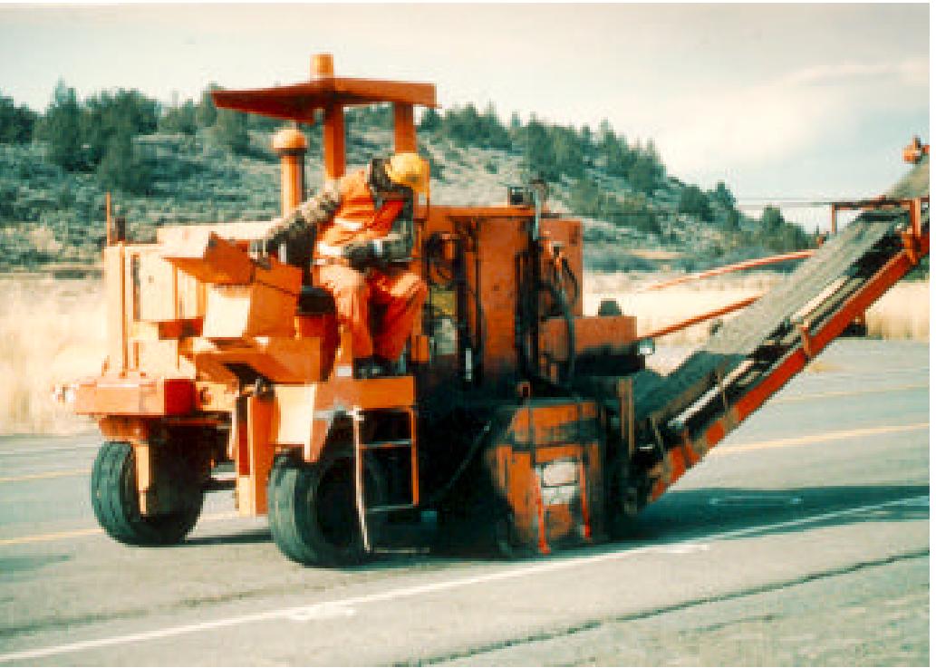
Figure 4. Semi-permanent procedure—straightening edges using cold-milling machine.
