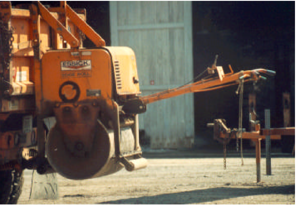
Figure 6. Semi-permanent procedure—single-drum vibratory roller used for compaction.
